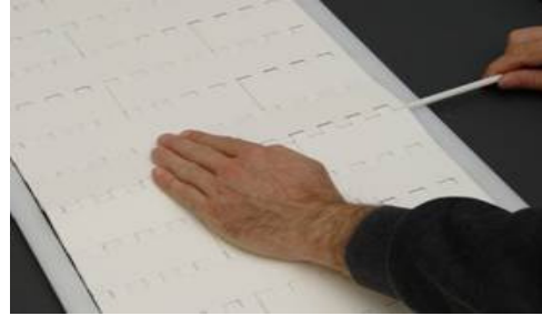
Insert rod For easy installation rod end must be beveled.
